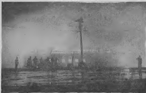
The flames were at their height when this picture was taken. The interior of the building that housed the bowling alleys has already been gutted and the roof is ablaze. See page 4.
